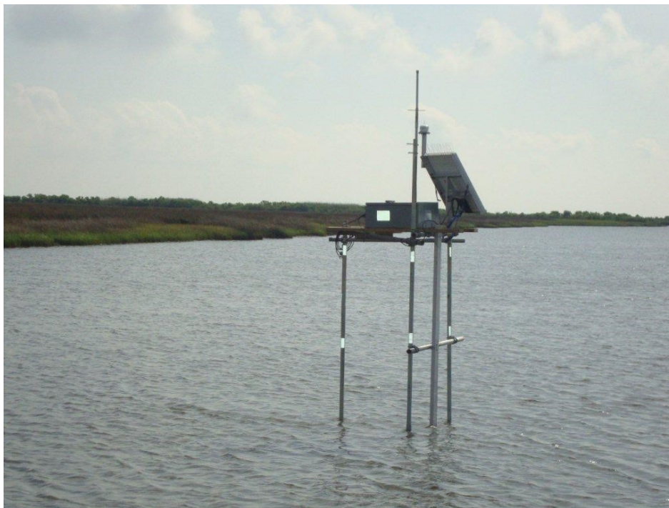
Figure 4. Image of the ADV platform type to be installed by USACE staff.
