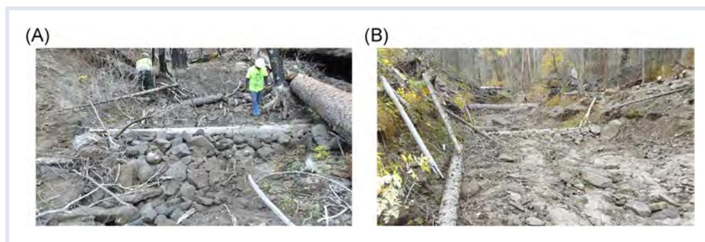
FIGURE 6 Sasquatch Canyon Erosion Control Structures—rock and lateral tree grade control structures to dissipate energy and stabilize the channel bed and banks
