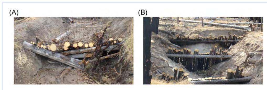
FIGURE 5 Switchback Canyon tree check dam erosion control structures designed to slow water and stabilize the channel
